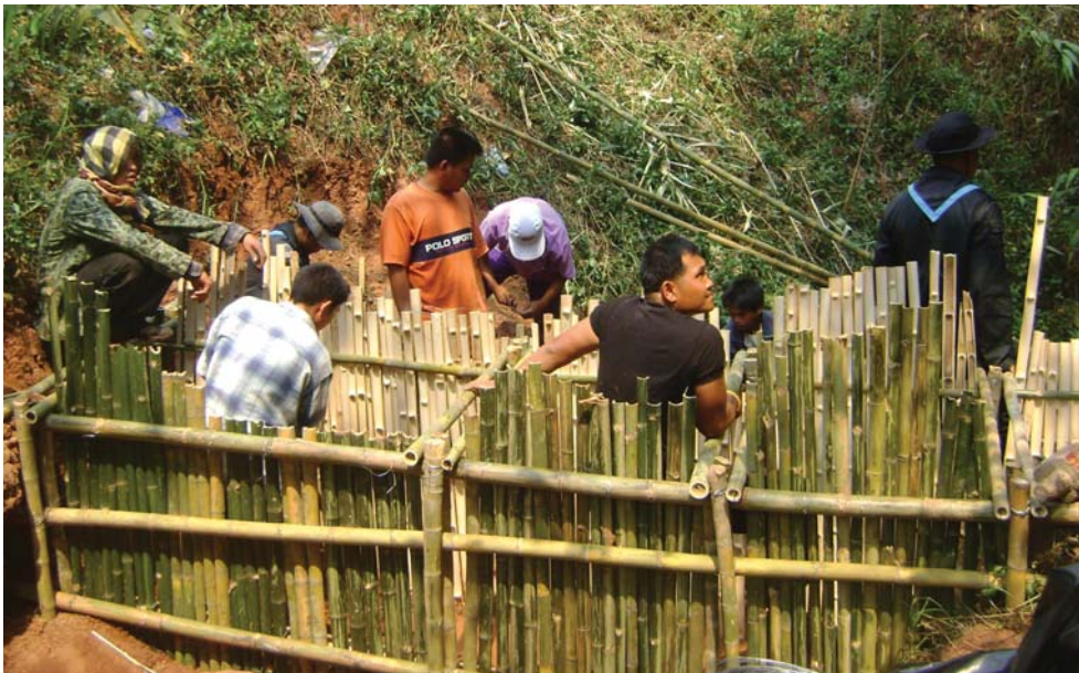
Figure 40: Fixing the laths into the ground
