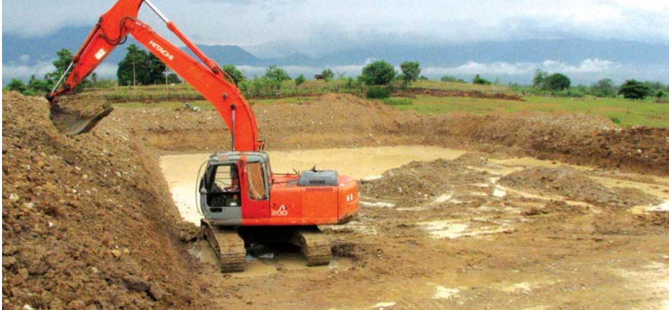
Figure 146: Levelling the surface of the construction site
