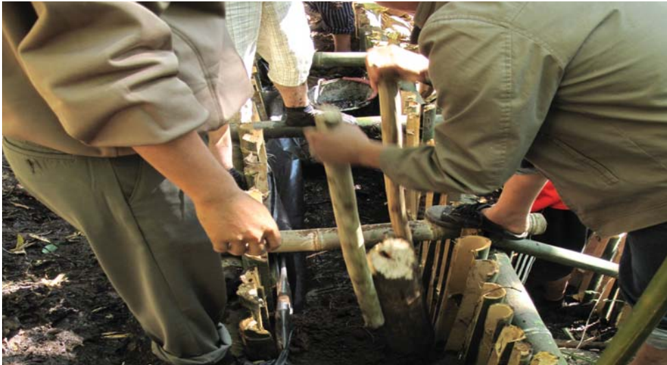
Figure 47: Compacting the soil
