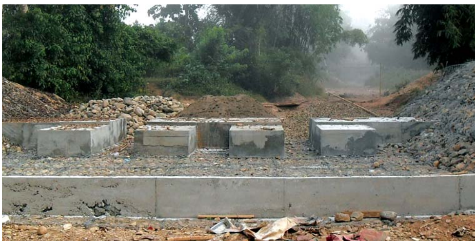
Figure 108: Gabions with partial concrete lining
