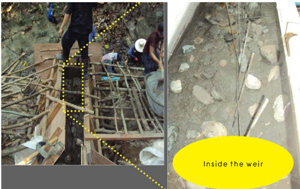
Figure 116–117: Leave rocks on the surface of the concrete if a pause is needed
