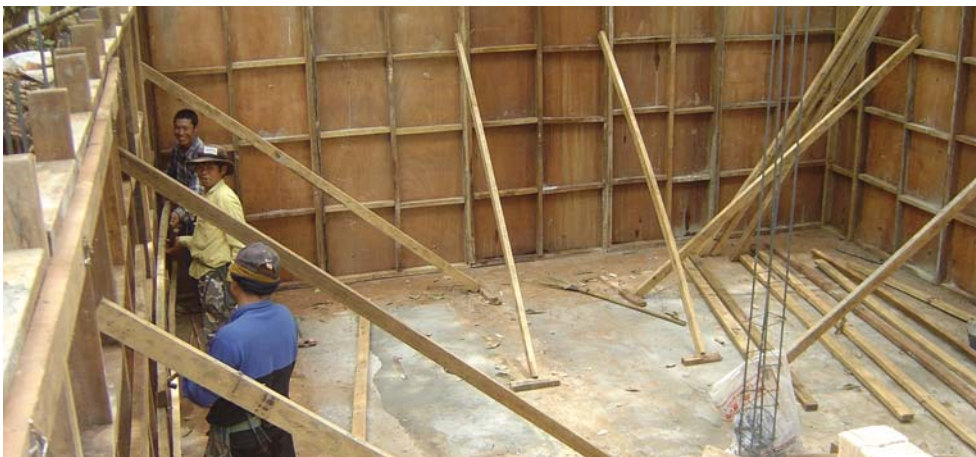
Figure 151: interior concrete form bracing
