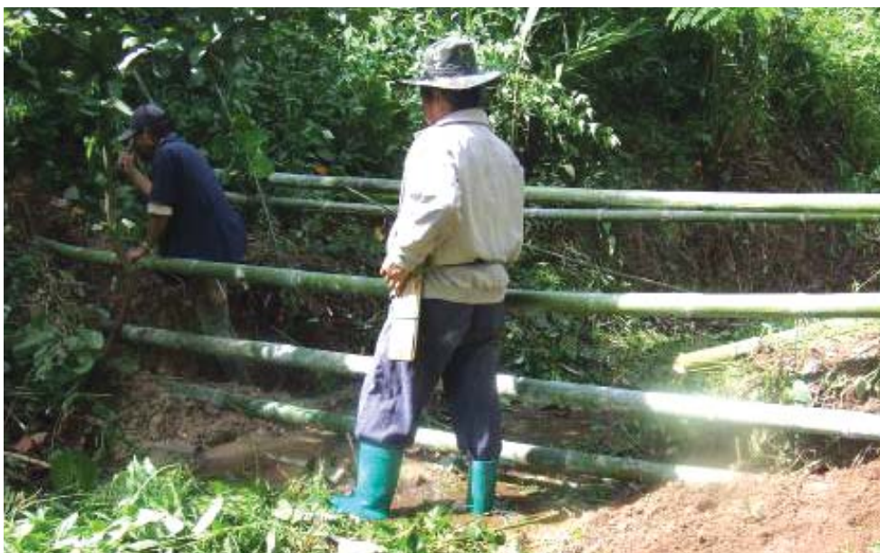
Figure 30: Placing the brace 1 metre apart
