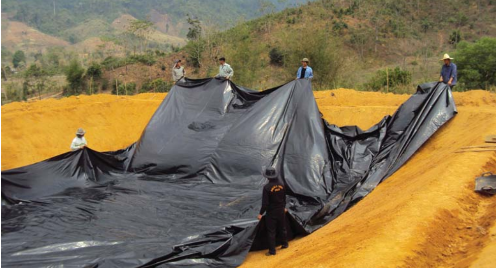
Figure 159: Opening the plastic sheet at the bed of a reservoir
