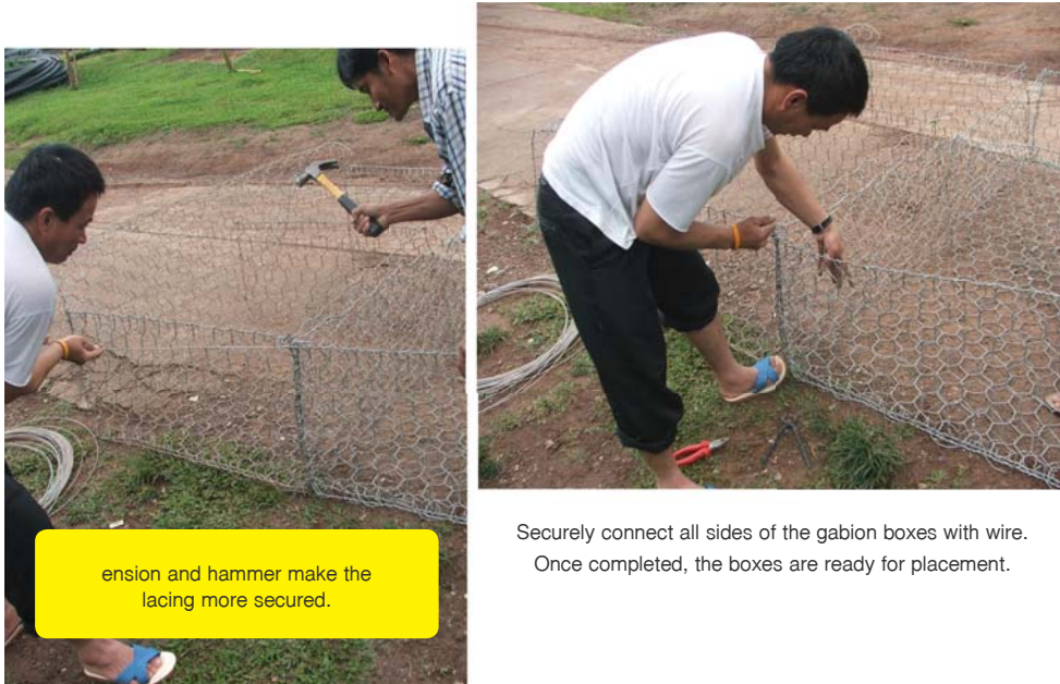
Figure 90-91: Completing the lacing process
