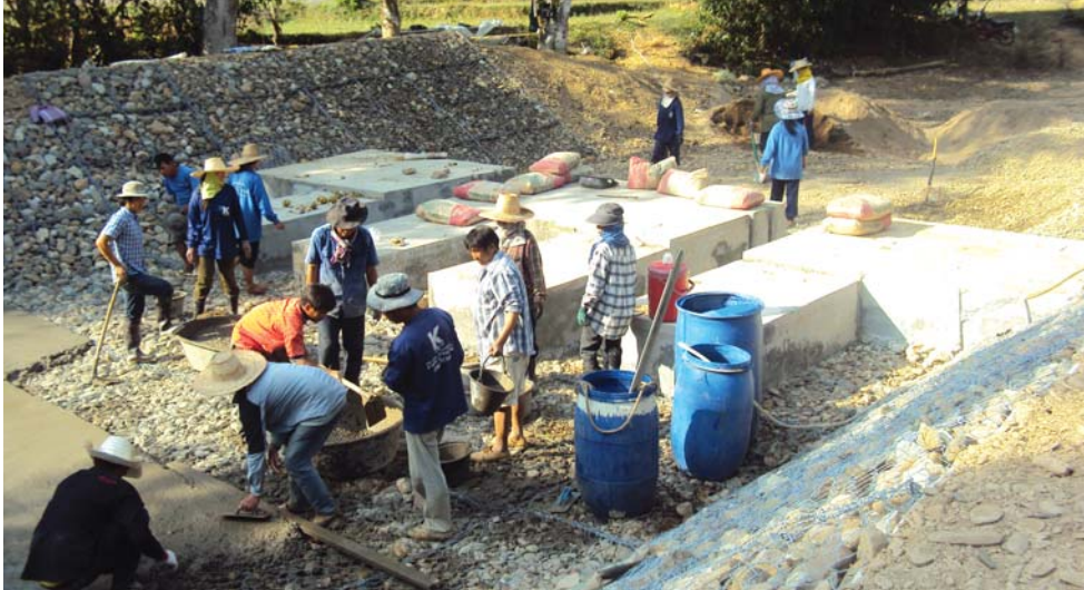
Figure 109: Gabions with full concrete lining
