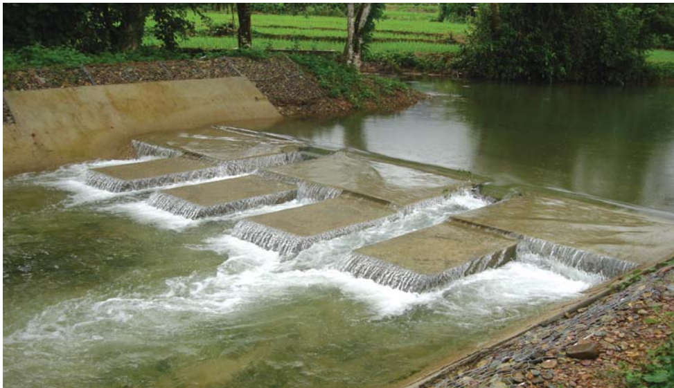
Figure 112: A completed gabion weir
