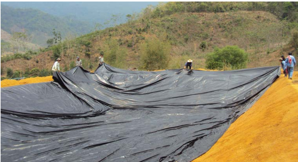
Figure 160: Spreading the plastic sheet over the reservoir structure
