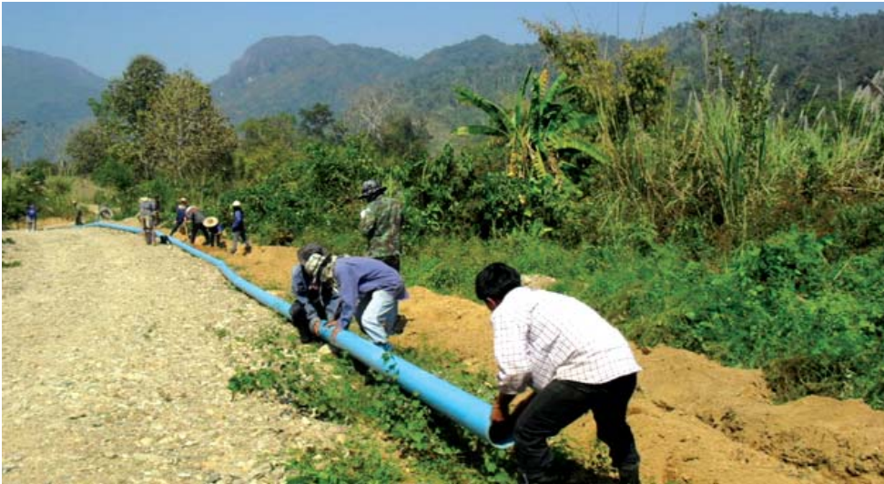
Figure 135: Placing pipes near the designated pipeline.
