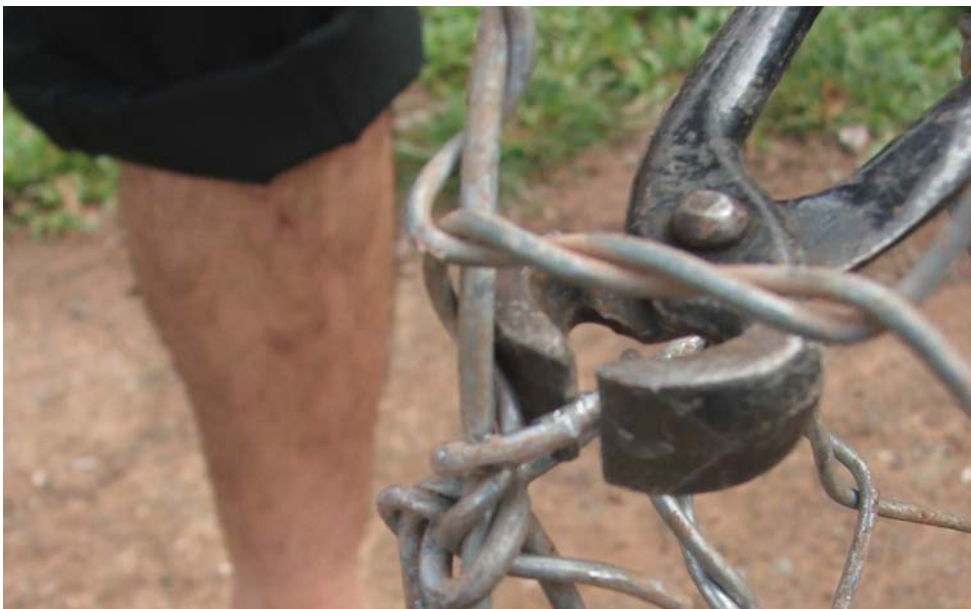
Figure 69: Lacing the edge of a gabion box
