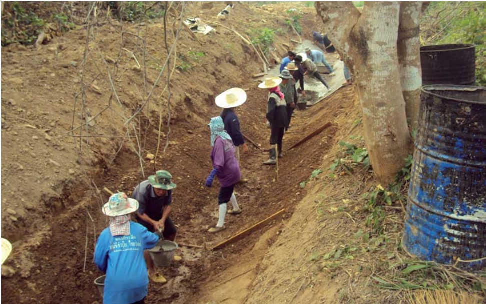
Figure 141: Concrete forms placement
