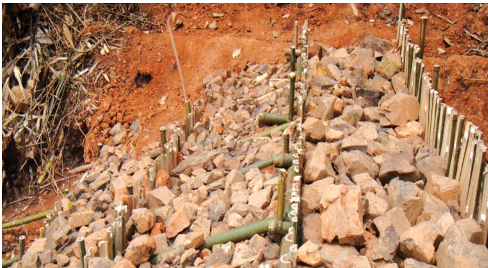
Figure 50: Check dam with rock cover
