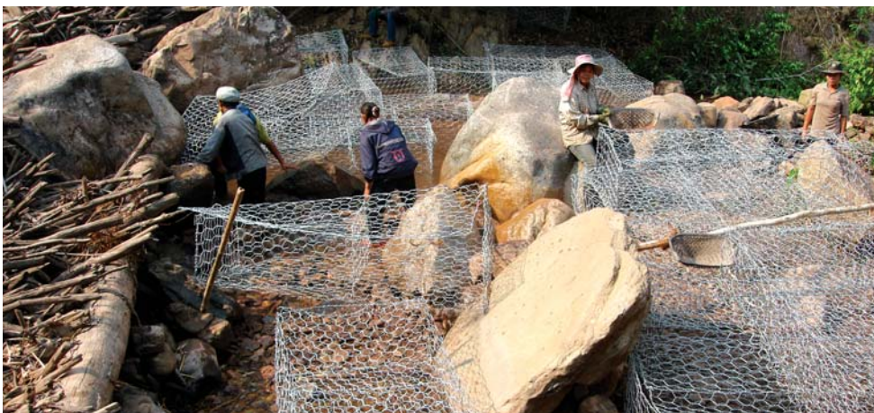
Figure 97-99: Placement of gabion boxes in the site with large rocks
