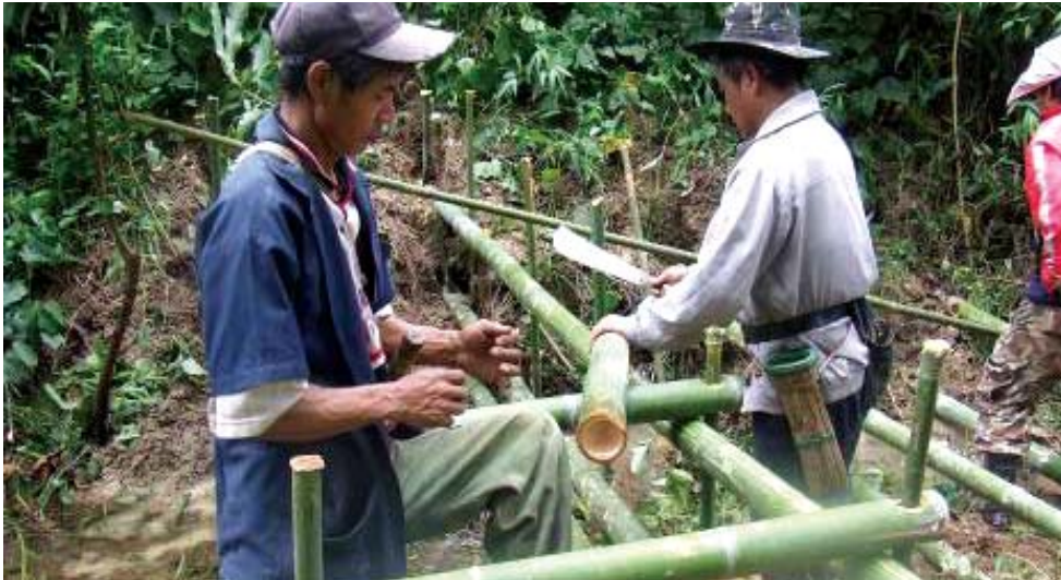
Figure 35: Placing joists over the posts
