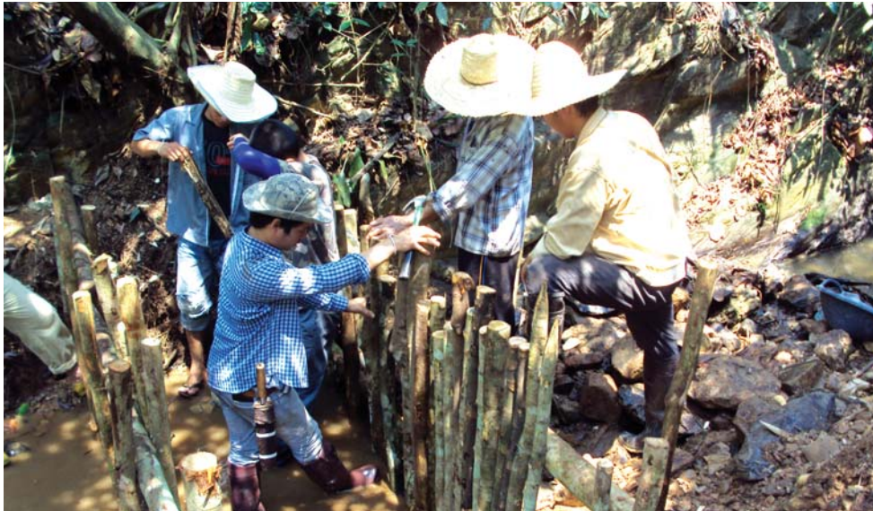
Figure 41: Putting up walls made of wooden laths
