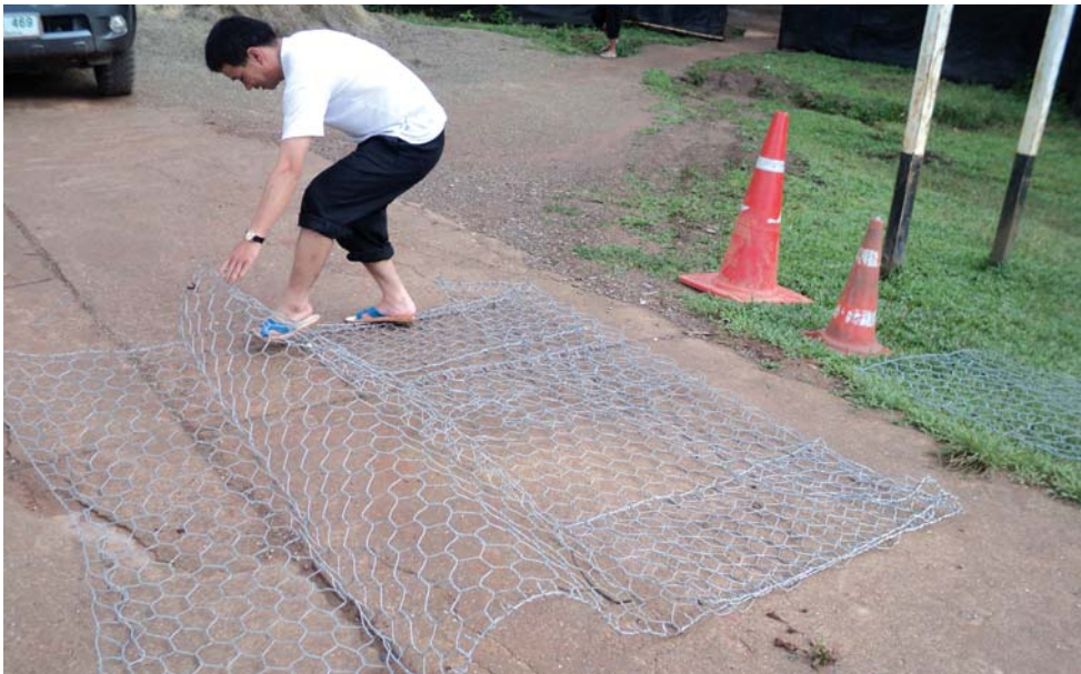
Figure 63: Unwinding the mesh
