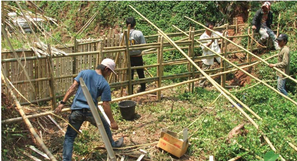
Figure 37: Placing rafters
