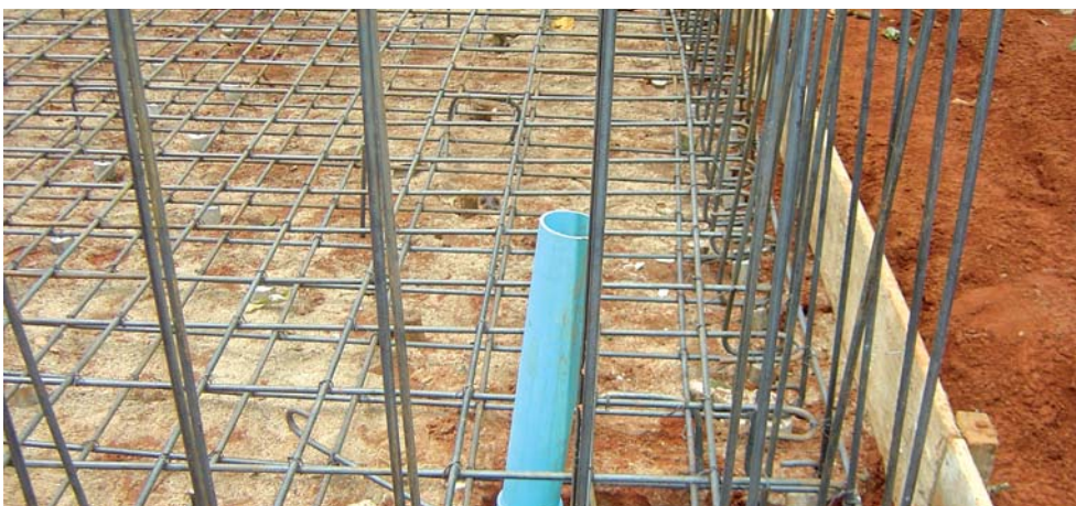
Figure 147: Concrete spacers, rebar formworks, and washout valve placement
