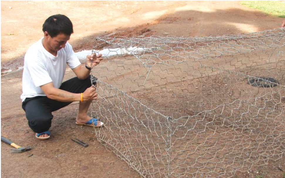
Figure 68: Lacing the edge of a gabion box
