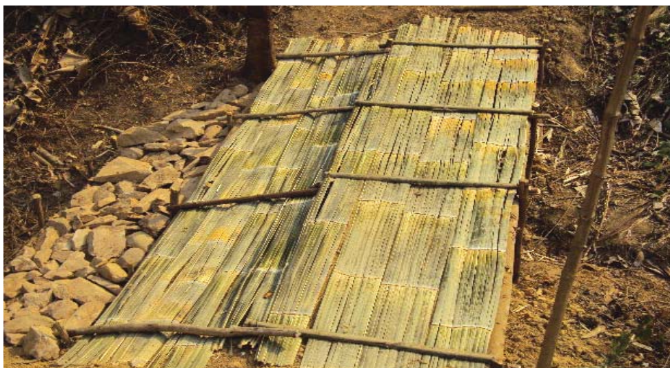
Figure 51: Check dam with a combination rock and bamboo cover
