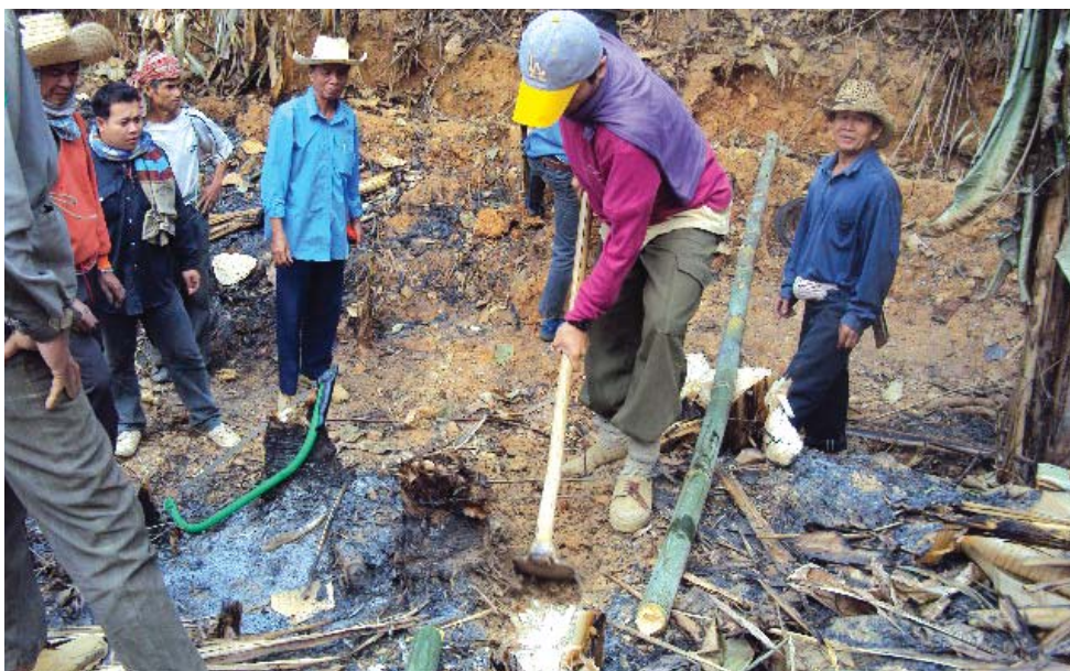
Figure 29: Digging a trough to place the braces.
