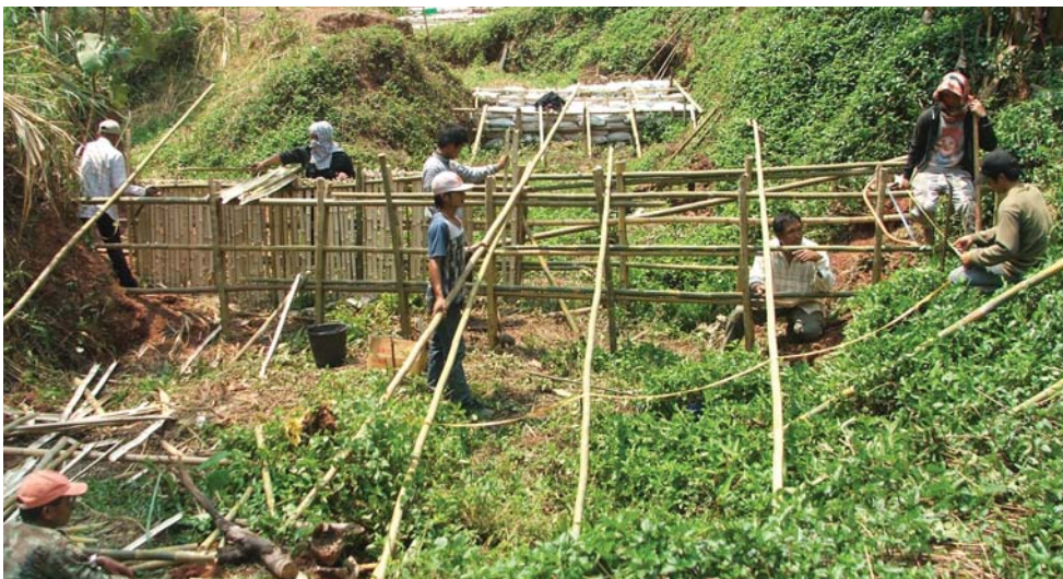
Figure 36: Placing rafters
