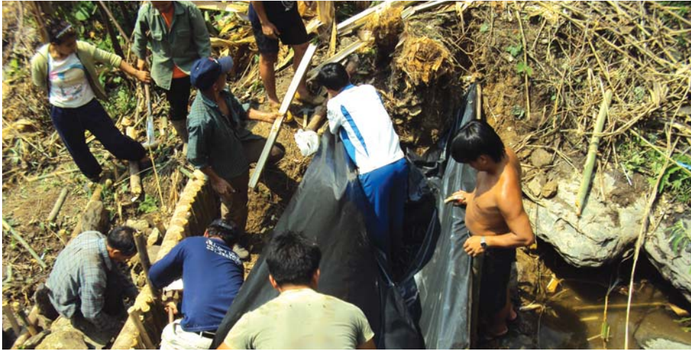
Figure 43: Installing the plastic sheet lining
