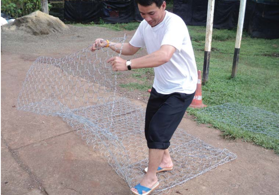
Figure 62: Unwinding the mesh
