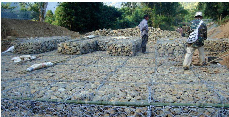
Figure 107: Gabions before concrete lining
