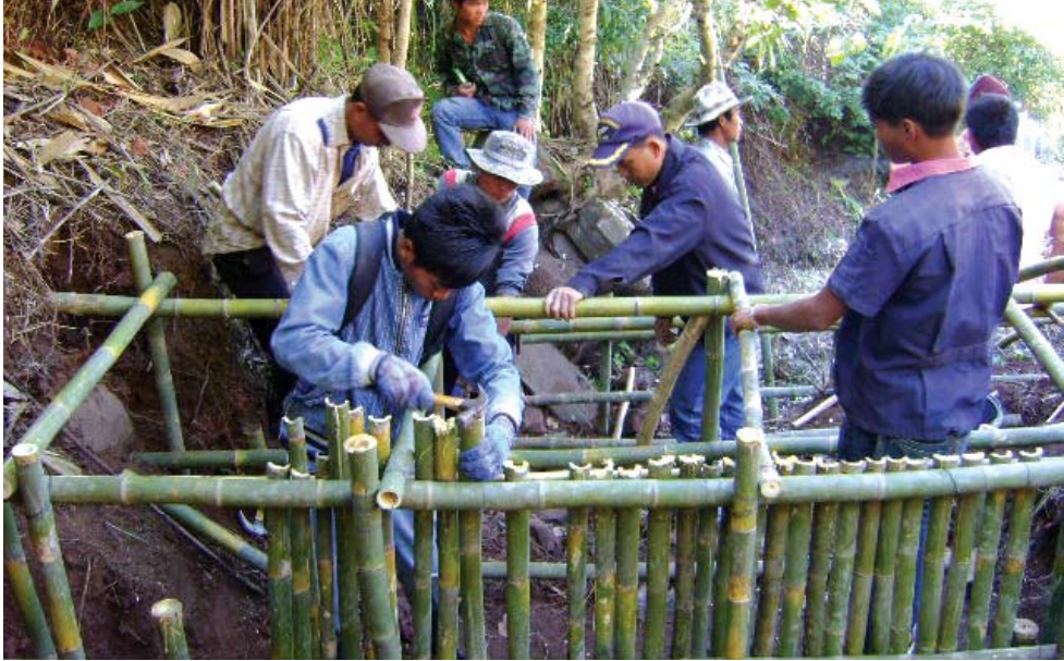
Figure 39: Fixing the laths into the ground
