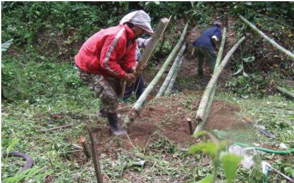
Figure 31: Securing the braces
