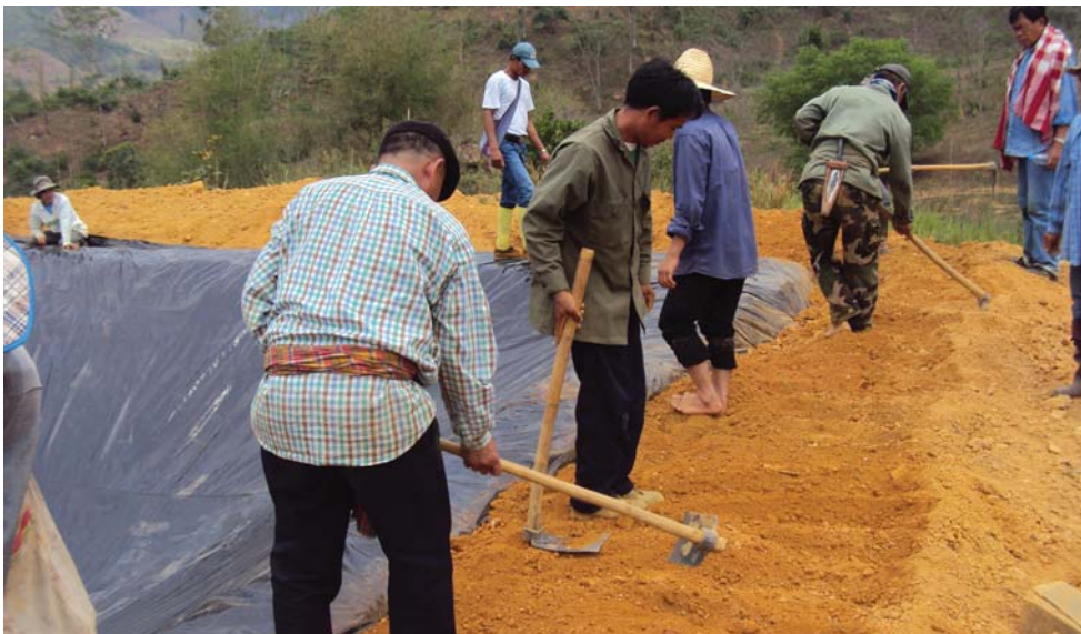
Figure 162: Backfilling the trench
