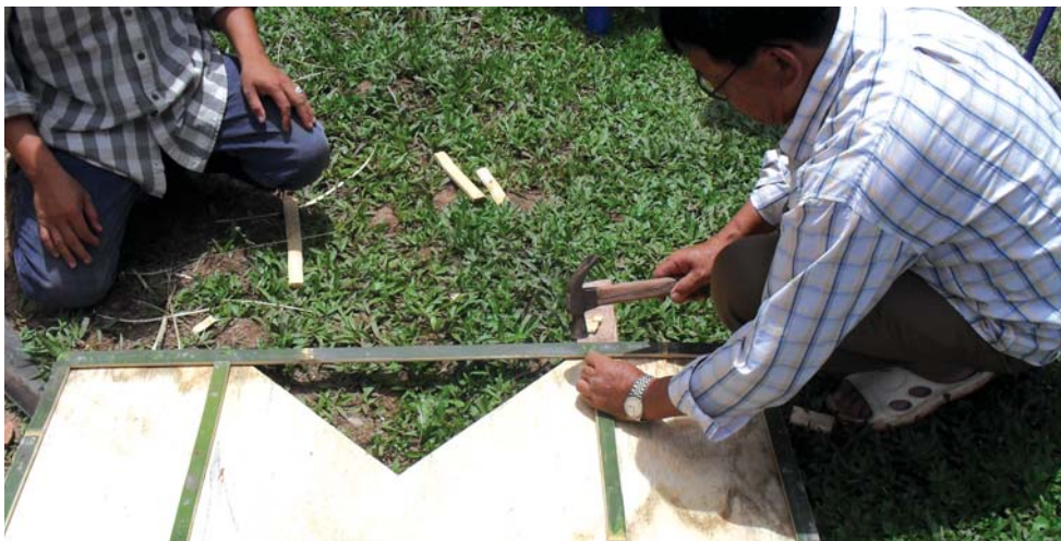
Figure 15: Reinforcing a V-notch plank with bamboo and nails
