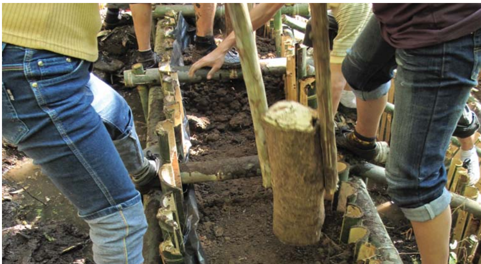
Figure 48: Spare a space of 20-30 cm height from the crest and fill it with large rocks
