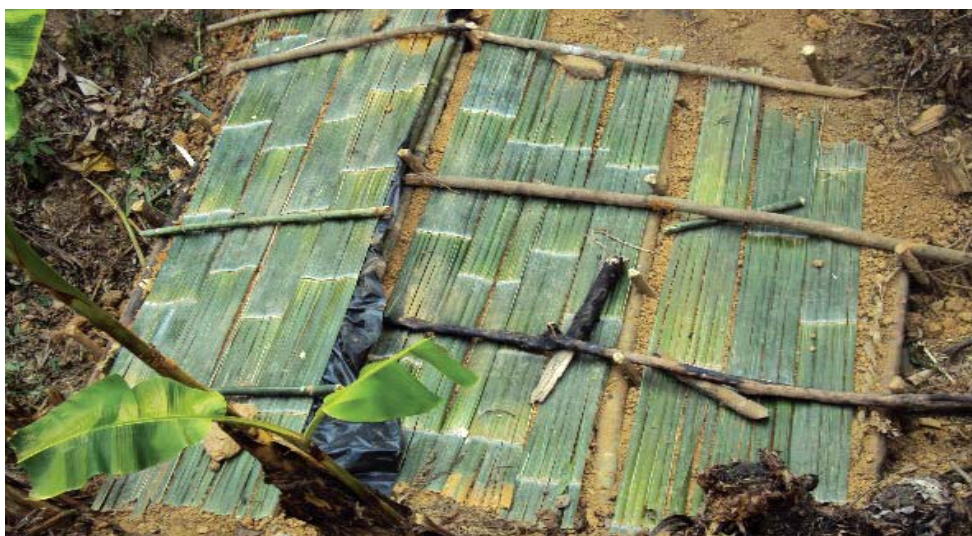
Figure 52: Check dam with bamboo cover
