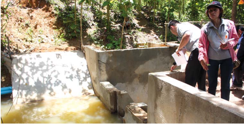
Figure 121: A reinforced concrete weir
