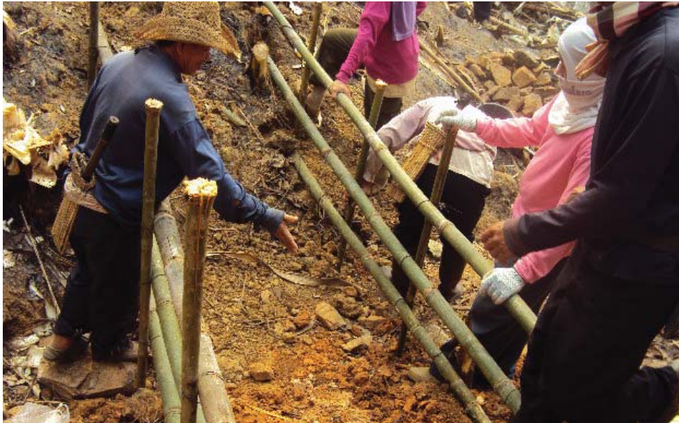
Figure 32: Hammering posts into the ground
