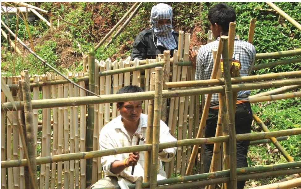
Figure 33: Securing the posts and braces together
