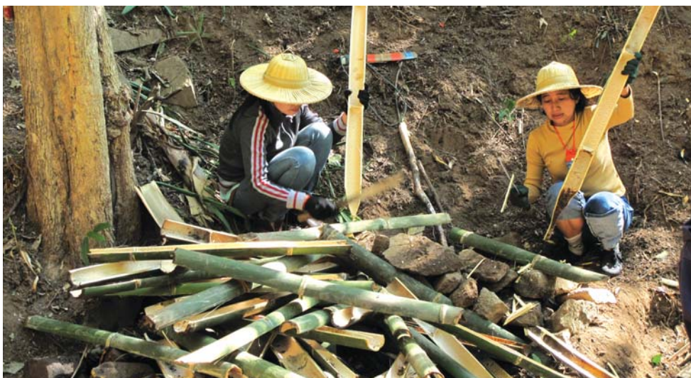
Figure 38: Cutting the bamboo tubes into half and use them as laths
