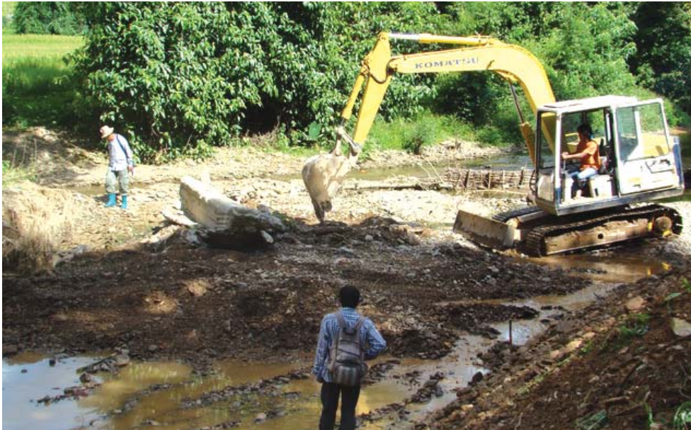
Figure 58: Preparing the site with heavy machinery
