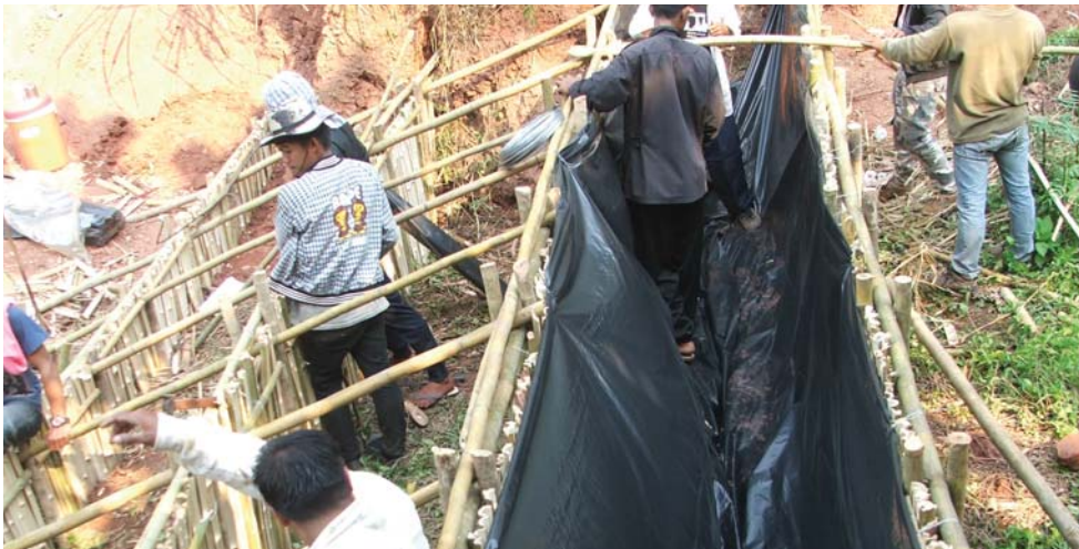
Figure 44: Installing the plastic sheet lining
