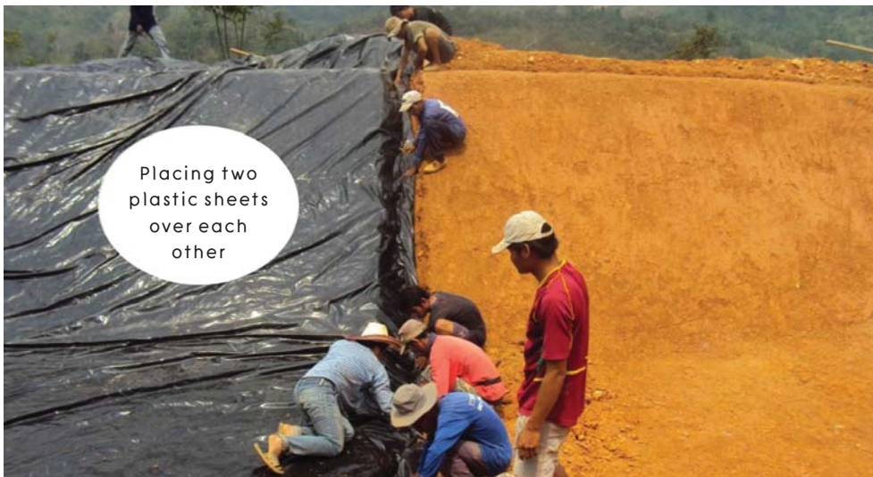
Figure 166: Securing the plastic sheet in the trench
