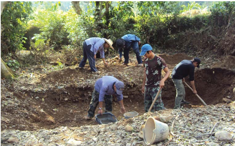
Figure 59: Manual site preparation
