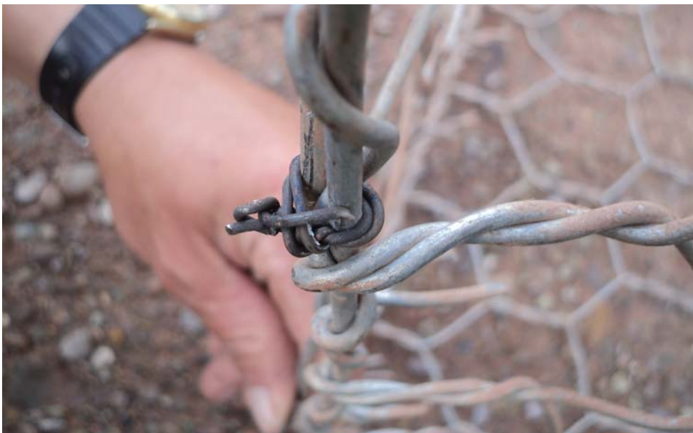
Figure 67: Double lacing each edge to retain the shape and strengthen the box
