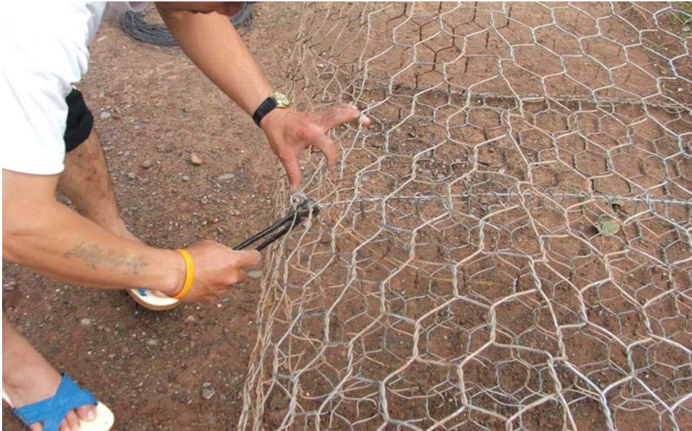
Figure 66: Lacing the edge
