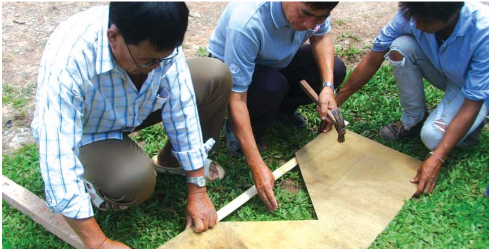
Figure 14: Strengthening a V-notch plank
