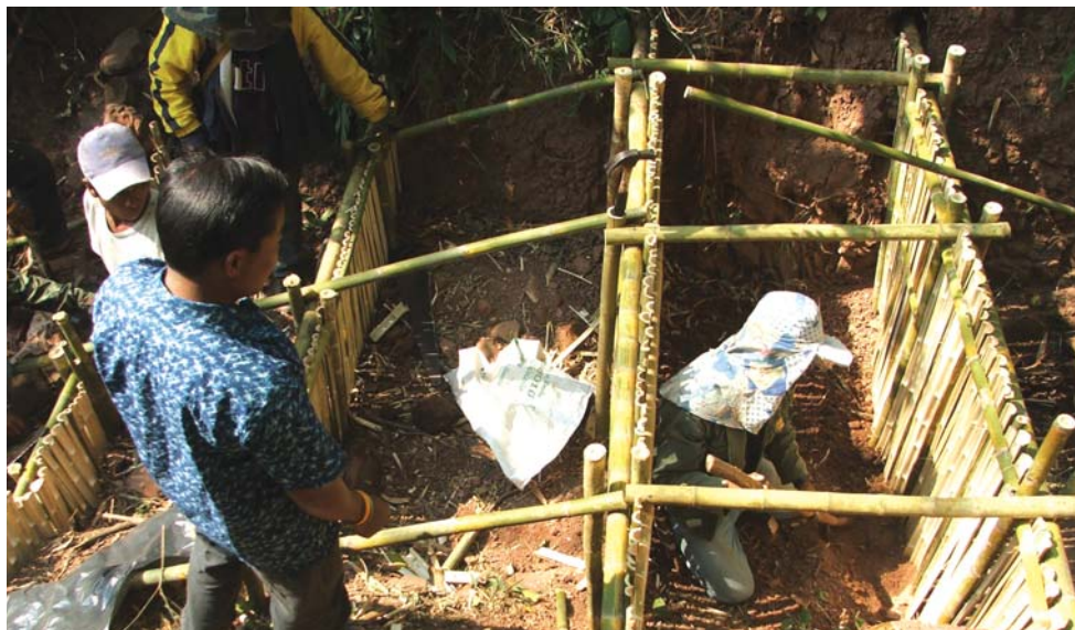
Figure 42: Digging a core trench
