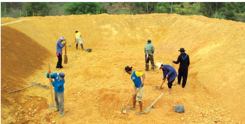
Figure 155: Clearing away unwanted rocks and debris from the site
