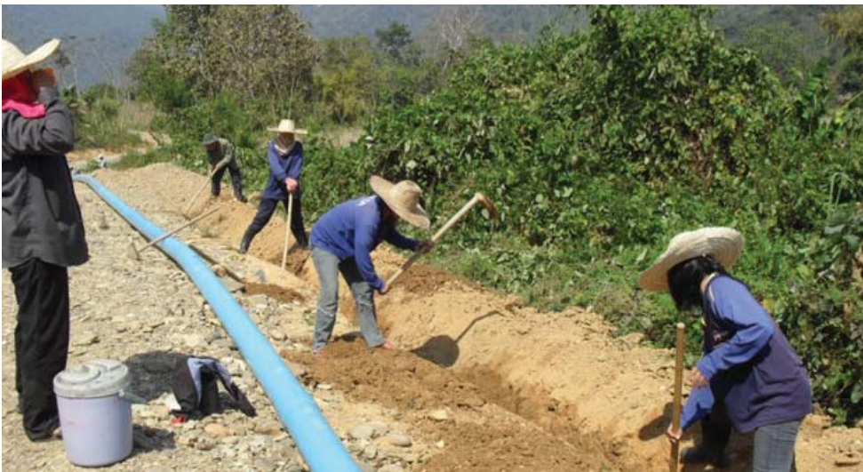
Figure 136: Trench construction
