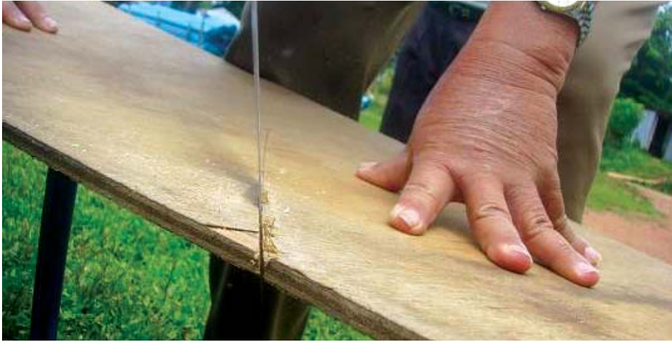
Figure 12: Cut plywood at 45 degrees
