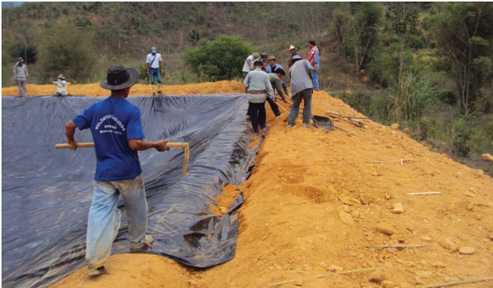
Figure 161: Film placement into the excavated trench
