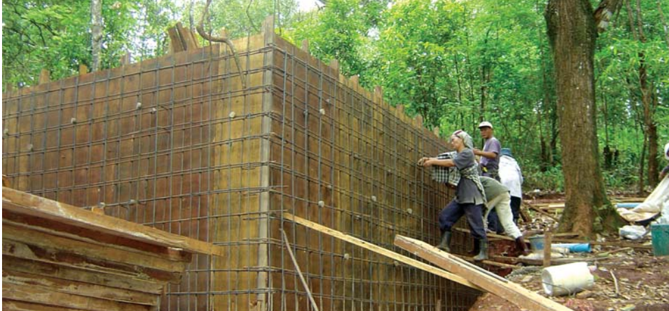
Figure 150: Exterior concrete form bracing
